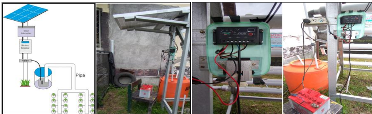
Figure 4. Solar power station component installation circuit
